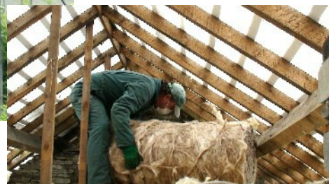
Ray busy laying the fibreglass in the attic.
