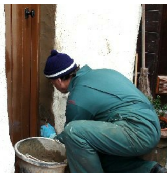
Ray finishing off around the door.
