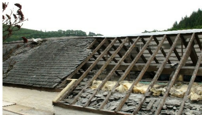
The old slates definitely were ready to be replaced.
