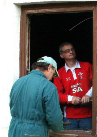
Dismantling the old living room window ready for the new.
