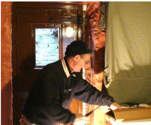
Left:- Brian busy fitting one of the doors
