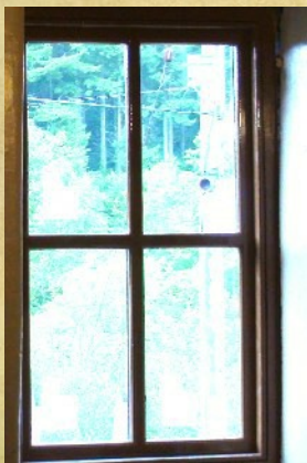
A new upstairs window.
