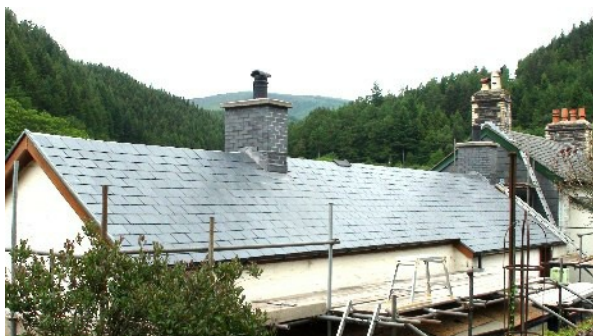
The finished roof and doesn't it look marvellous. Ray shouldn't have to go up there again to fix any fallen slates.
