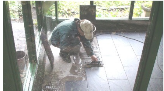
Ray laying the slate tiles.
