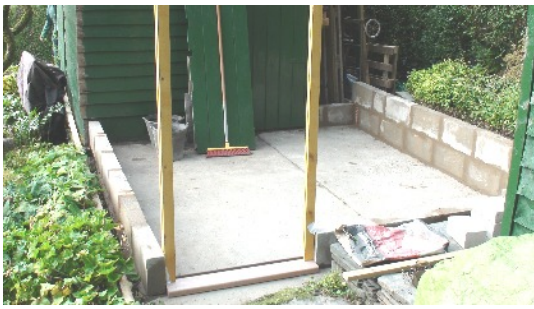
It was so exciting, the first few blocks were laid and I helped Ray to point them.
