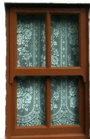
A newly fitted downstairs window, I think it looks great, so in keeping with our cottage. Plastic ones would have been hideous.
