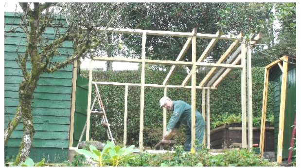
The frame work being built, carpentry is Ray's favourite DIY task..
