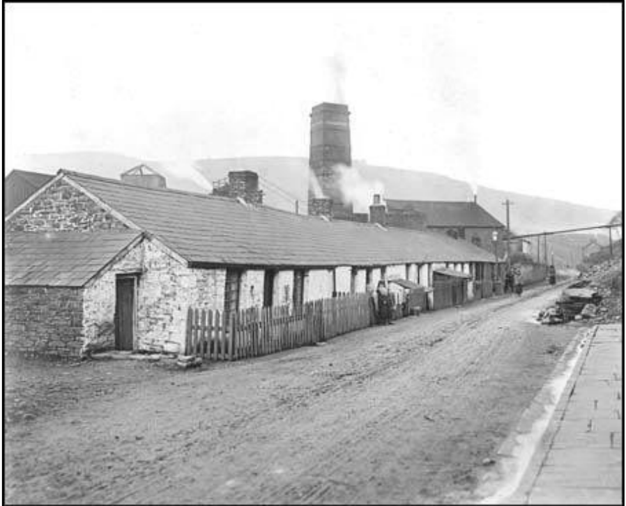
The Cymmer colliery cottages, built in the early days for colliers of the company
