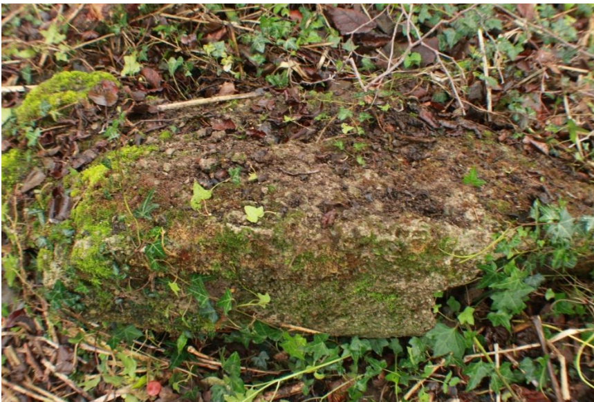
Ffigur 7 / Figure 7. Cymraeg: Bloc sylfaen carreg sylweddol wedi'i leoli ger lan yr afon, gyda mortar tebyg ei gyfansoddiad i'r mortar a welir yn wal amddiffynnol yr afon, ond gyda gwead mwy trwchus a chryno. Gellid dehongli'r bloc hwn fel rhan o sylfaen colofn neu strwythur cynhaliol, wedi'i leoli tua 80 m i'r de-orllewin o wal yr afon. English: Substantial stone foundation block located close to the riverbank, bonded with mortar similar in composition to that observed in the river defence wall, though denser in texture. This block may represent part of a column base or supporting structure, situated approximately 80 m south-west of the river wall.
