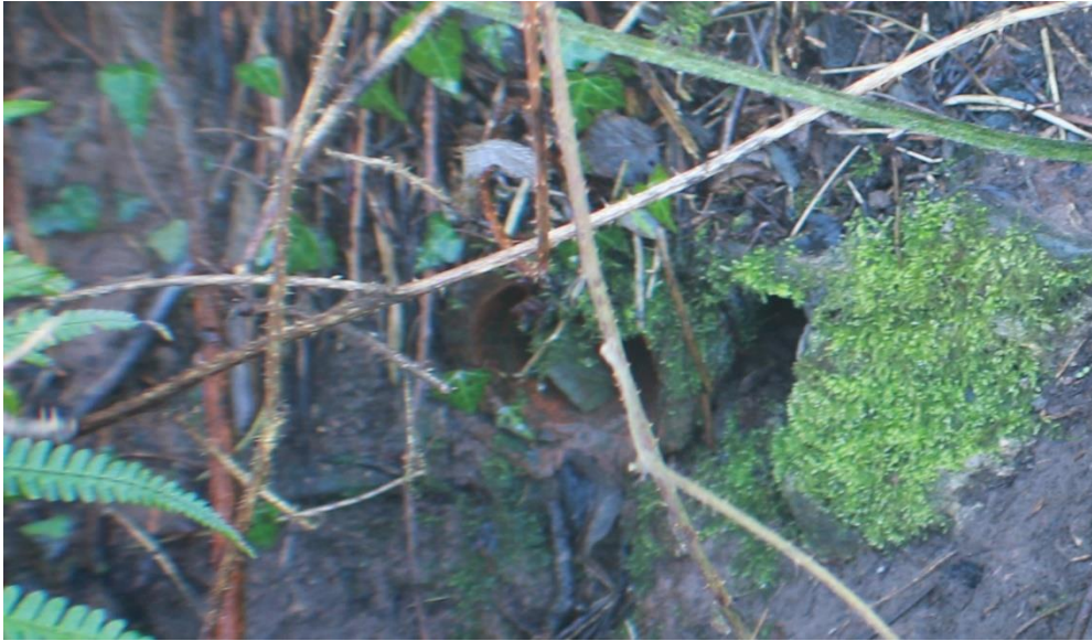
Fig 15/16 (15) Showing drainage pipes possibly from the bathhouse C that serves the amphitheatre. The pipes are clear SE to the amphitheatre server road. Coordinates: 51.56917, -3.10962
