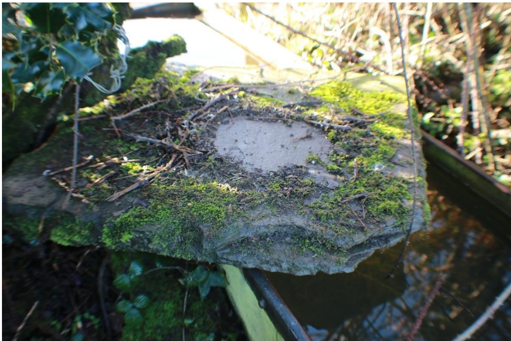
Fig 19/20/21 (20) Showing a possible paving stone or culvert cap stone at the bathhouse B position. Coordinates: 51.57054, -3.11147
