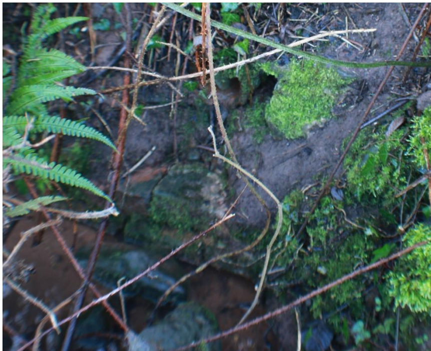
Fig 15/16 (16) Showing drainage pipes possibly from the bathhouse C that serves the amphitheatre. The pipes are clear SE to the amphitheatre server road. Coordinates: 51.56917, -3.10962
