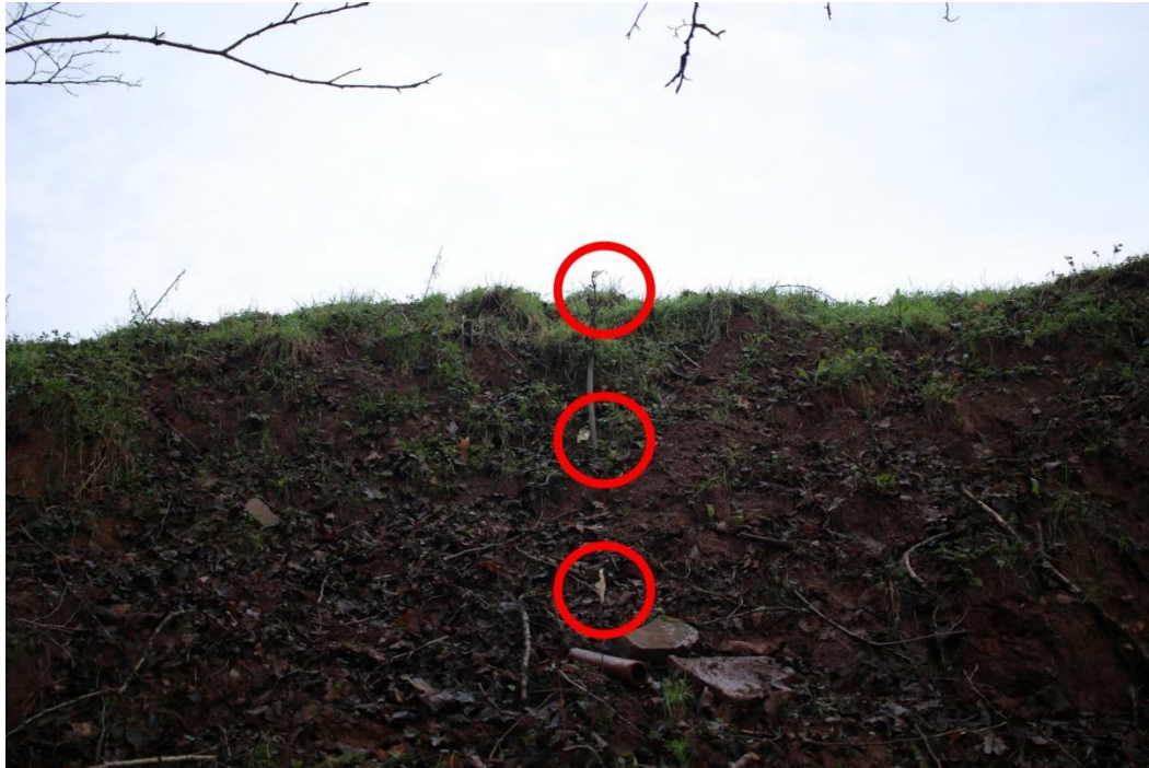
Fig 28//29 (29) Showing the exercise channel edge's, approx 10/11 m width. Also showing it depository position terminal to drainage waterway. Coordinates: 51.56605, -3.11533
