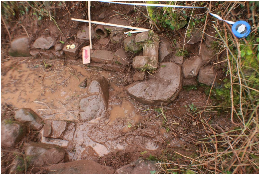
Figure 25: Masonry remains in waterway
