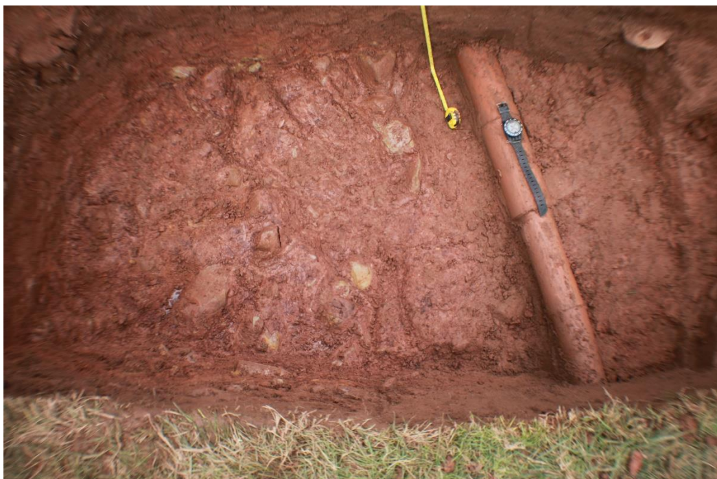
Figure 3A: Trench 1 extended west showing foundation stone adjacent to drain pipe and road correlation.
