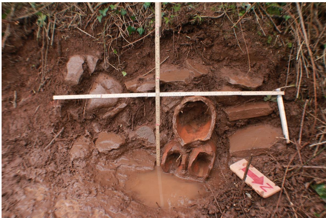
Figure 8: Triple ceramic pipe drainage terminal exiting the waterway bank with measurement scale.
