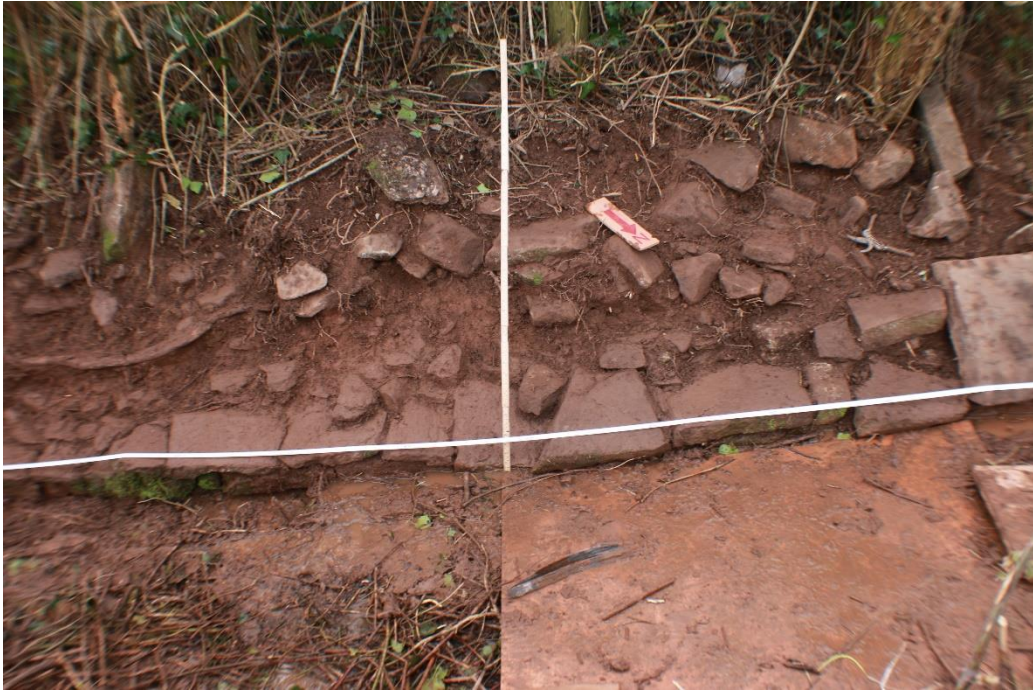
Figure 6: Road support structure and bearing stones.
