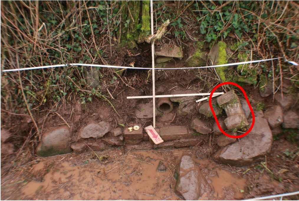
Figure 24: Masonry remains in waterway
