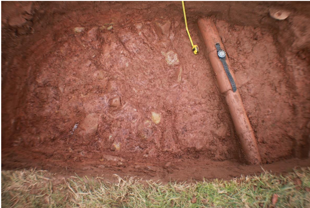
Figure 3A: Trench 1 extended west showing foundation stone adjacent to drain pipe and road correlation.
