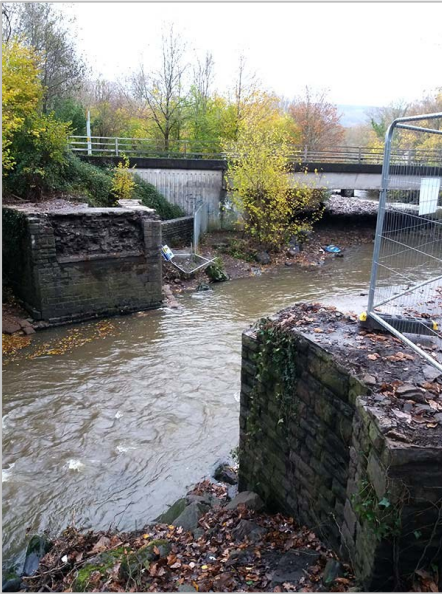
When the bridge deck had been removed.
