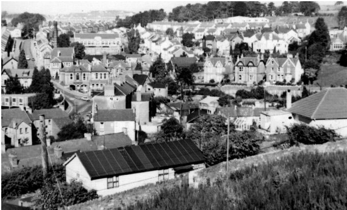
The “hut” in Penyard as seen from The Avenue [photograph Martin Conisby]
