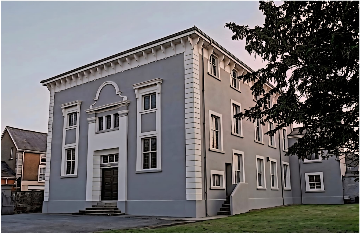
Capel Sul (formerly Rumsey House), Bridge Street, Kidwelly. Built 1862 in Italianate style, this was the home of Harold and Mabel Greenwood at the time of her death in June 1919. Purchased by the Independent congregation in 1923 and converted to a chapel 1924–26. Digitally enhanced photograph by Graham Tudor Emmanuel, Tudor59, Kidwelly, 2026.
