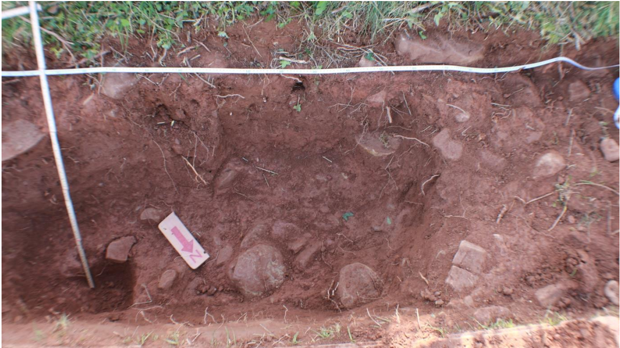
Figure 33: Detail of compacted base material within Trench 8, supporting interpretation of an engineered road foundation.
