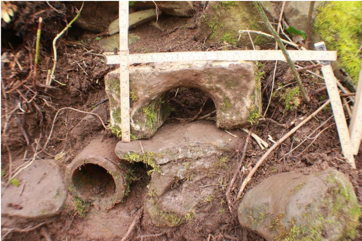
Figure 27: Bath stone arch block
