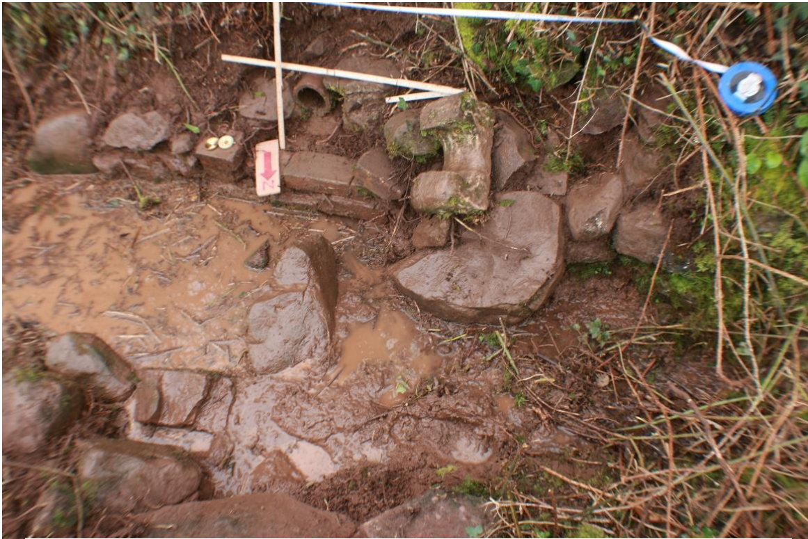
Figure 25: Masonry remains in waterway
