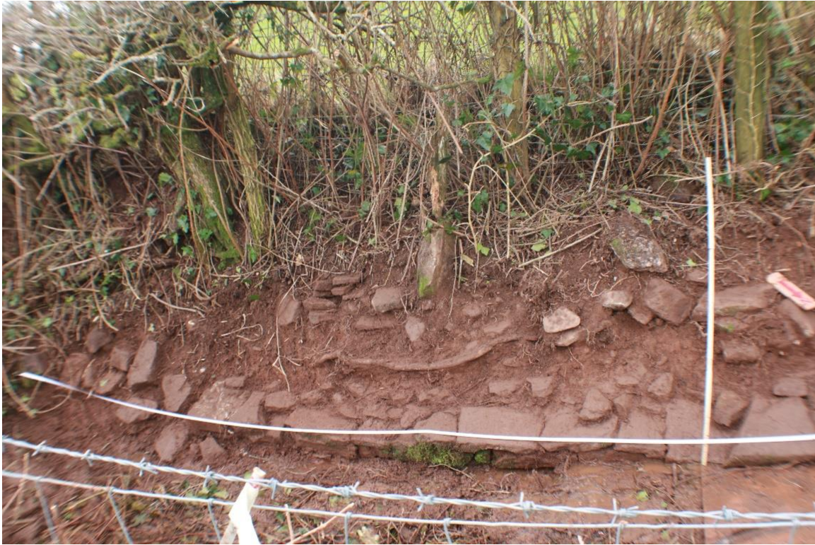
Figure 5: Exposed road face at waterway crossing showing roadside edge and metalling.
