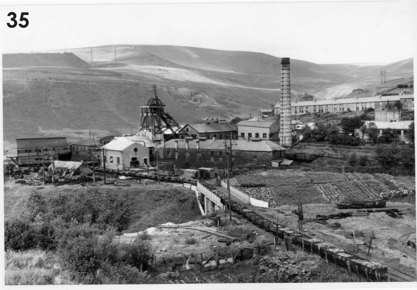
Wyndham/Western Colliery, 23 November 1954
