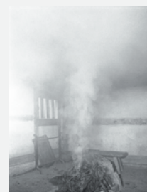
Without a chimney, the room could be smoky in the time of the Tudors.
