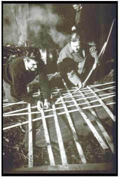
A Towy coracle is traditionally made from woven ash laths, held together in a basket weave with a woven hazel gunwhale. There are seven longitudinal laths and the same number of cross laths.
