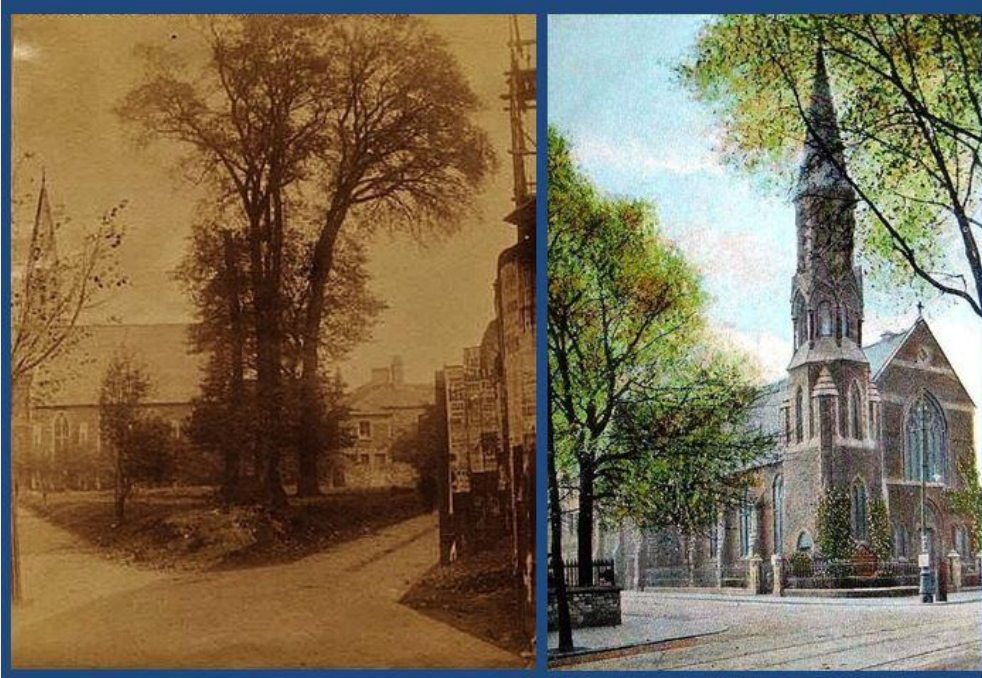
Clifton Street Presbyterian Church . Left: the original four elms with the church in view behind, before Roath library was constructed (photo: Cardiff Libraries)
