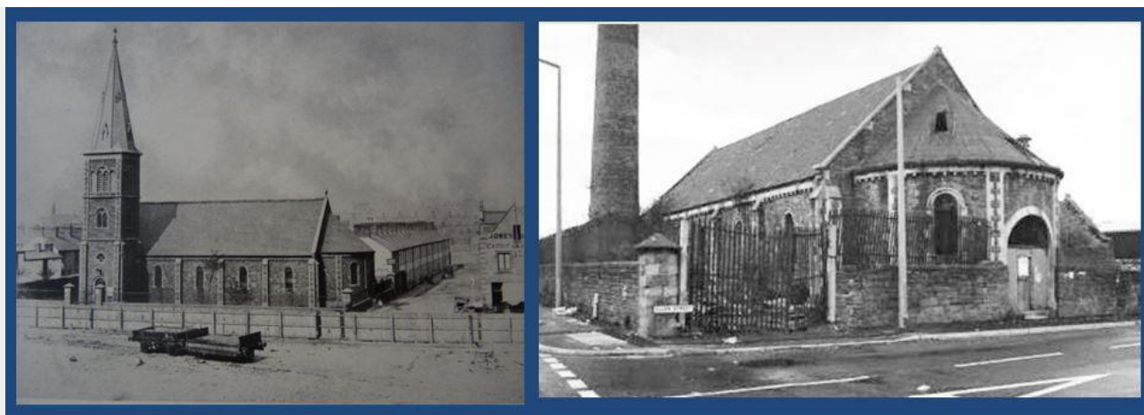
All Saints, Tyndall Street, Newtown, Cardiff. Rt: with spire demolished and replaced by a chimney.
