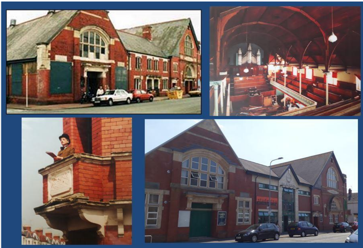
Crwys Hall. Top – the original buildings during renovation. Bottom left: a recreation of the exterior pulpit being used (photo credits: Tony Cort). Bottom Rt: Highfields Church.
