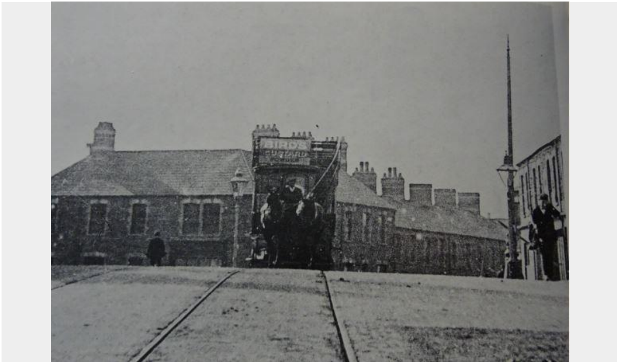
Splott Bridge looking towards Agate Street, 1902. St German's Mission, 18 Agate Street – obscured by the bus
