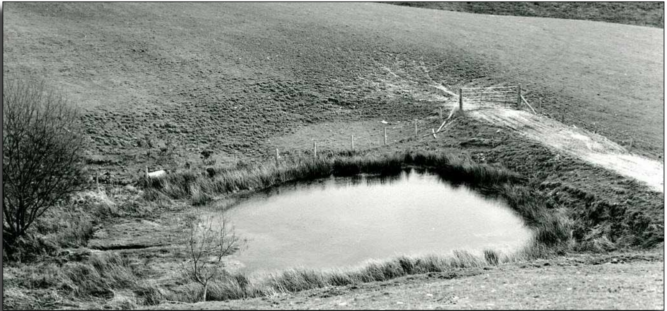
The upper reservoir built to supply power to Rhiwgreiddyn quarry, called Llyn-y-Mynydd.
