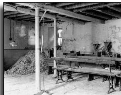
The vestry below the chapel in April 2001. Picture by Ray Gunn.
