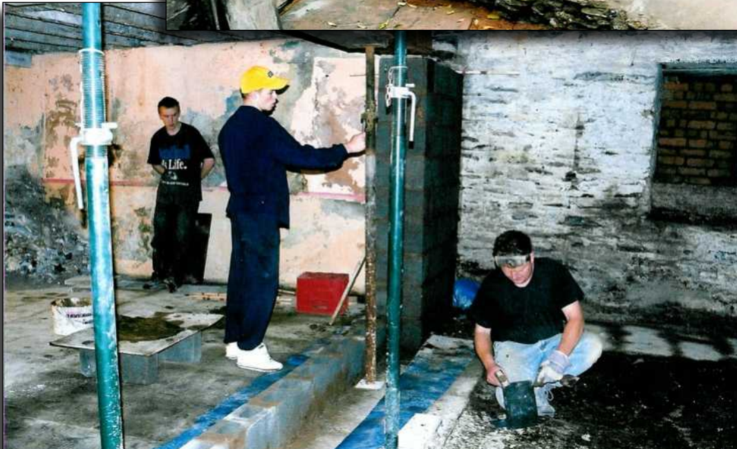
Michael Blackwell, left and Jeremy Andrews, right, working on the old vestry under the chapel, with the owner's son Jason Thomas, centre, 2001. Picture by Julia Gunn.
