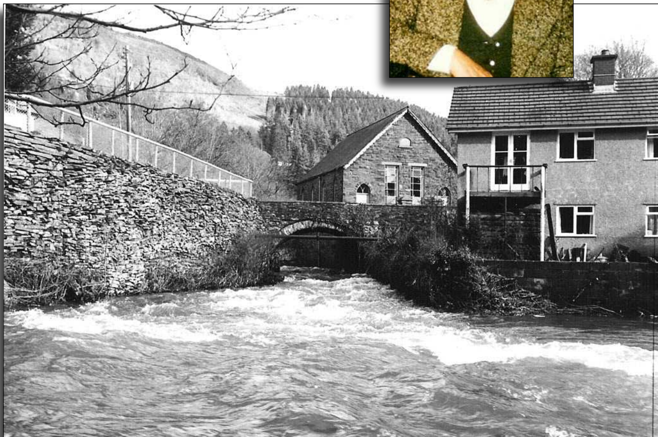
Aberglesyrch bridge, with Aberglesyrch cottage on the right and the Methodist chapel, centre, 1998.
