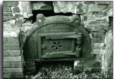
The furnace door under the enamelling ovens, dated 1884. Picture, 2000, by Ray Gunn.
