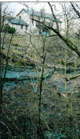
A rear view of Swn-yr-Afon, 2003, showing some of the landscaping work done by Owen Kirkham for the Dignams.
