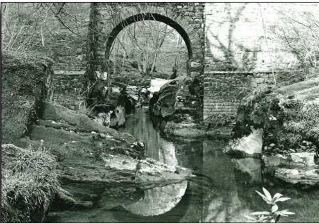
Evans bridge from downstream, 2000. There are further buttresses on this side built to strengthen the bridge in the 1970's. Picture by Ray Gunn.
