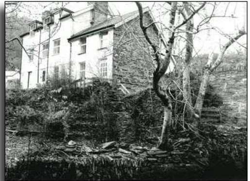
Below Dulas Cottages, showing the crumbling parallel walls of the old tramway bridge, 2003. Picture by Ray Gunn.
