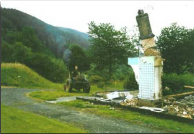
7 & 8 Heulfryn, the camp, being demolished in Aug. 1986, with Gerald Groom on the tractor. Picture courtesy Hugh Davies.
