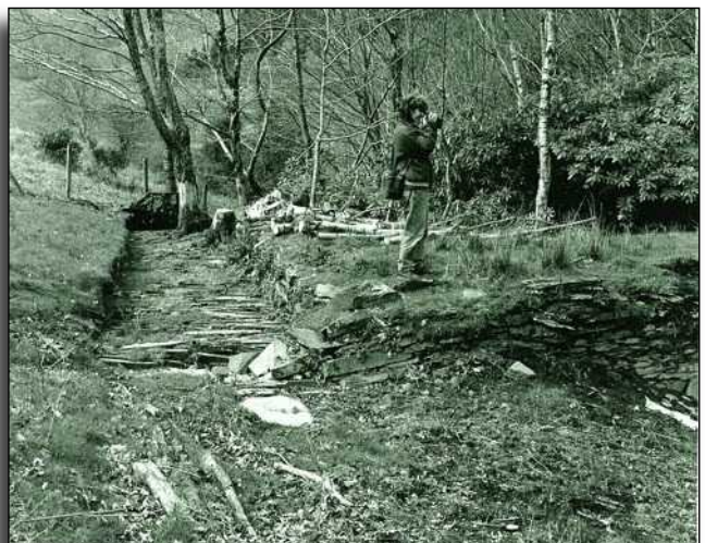
The overflow channel of the lower reservoir, neatly constructed in slate. The figure is Julia Gunn. Picture 2000, by Ray Gunn.
