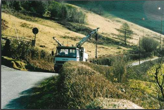
British Telecom erecting poles for the first time on the roadside South of the village, Jan 2003. Picture by Julia Gunn.
