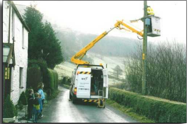
British Telecom connecting the new line to the new poles, 2003, watched by Louise Gunn & Connor, Kieran, & Cameron Jones. Picture by Julia Gunn.
