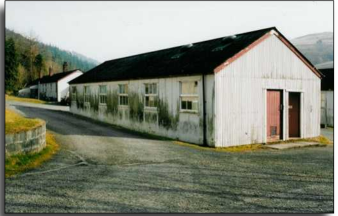
An old store with toilets at the near end for forest workers in the camp, 2003. Picture by Julia Gunn.
