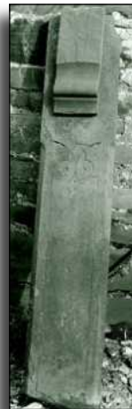
An example of the slate finishing work carried out at the quarry. Picture 2000, by Ray Gunn
