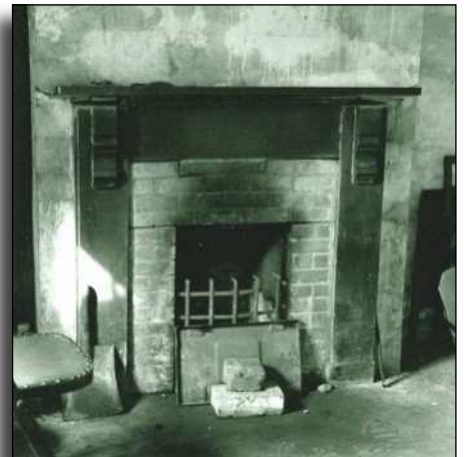
A fireplace in the old office at the quarry. The red slate surround was made and enamelled there. Picture, 2000, by Ray Gunn.
