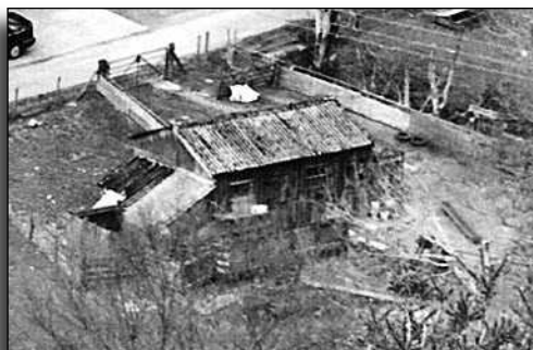
The farm buildings at Panteg, 2002. Picture by Ray Gunn.
