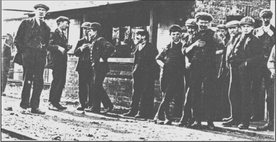
Colliers young and old outside the wages office. Date & colliery unknown
