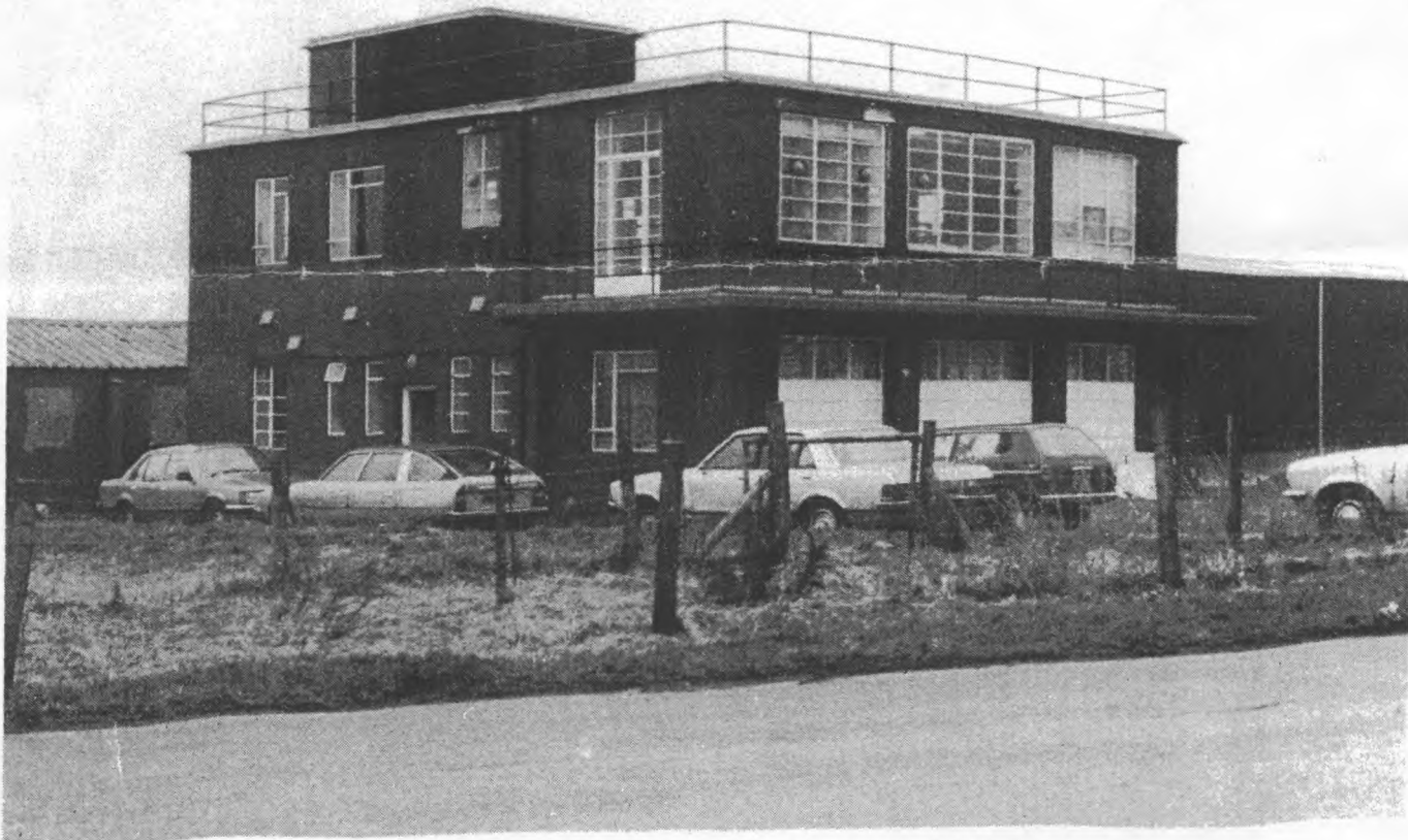
The control tower at Llandow, now used as offices, as seen in February 1982. Photo: Aldon P. Ferguson
