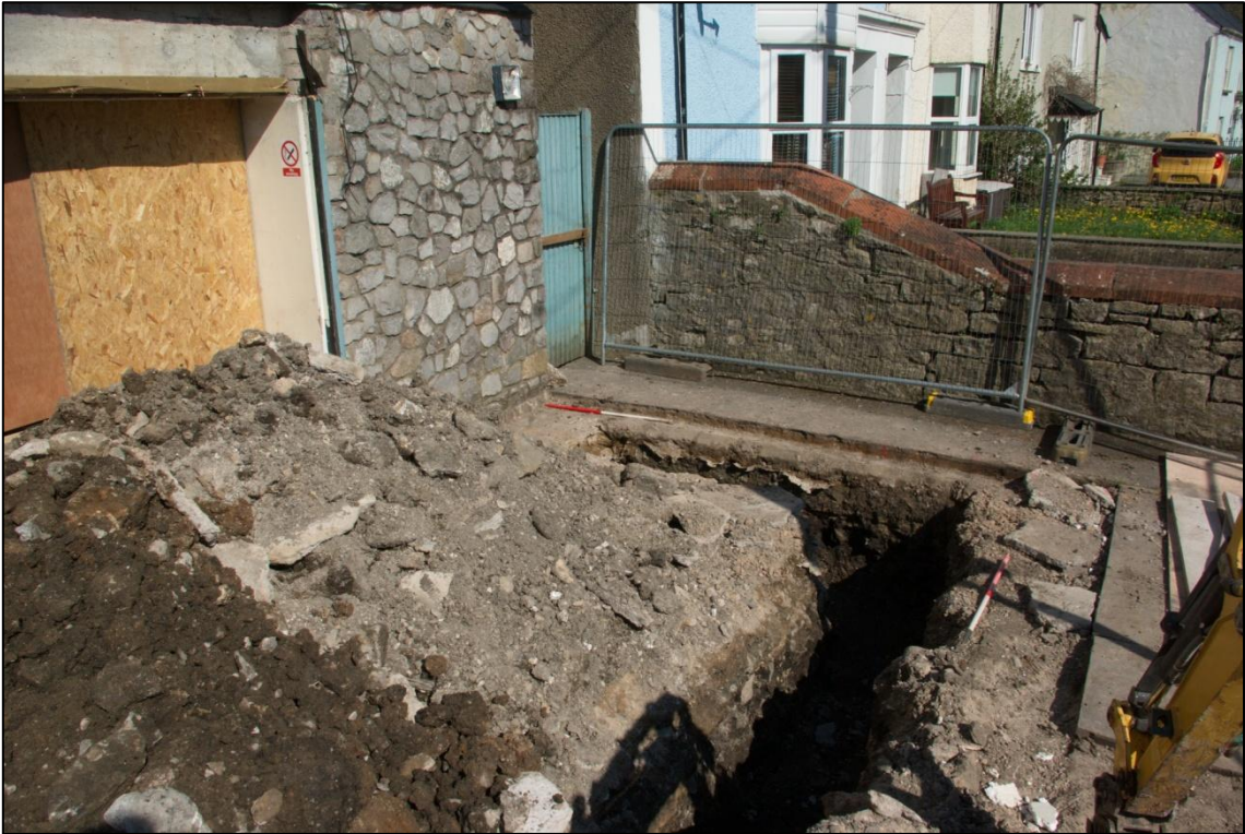
Plate 1: The watching brief area from the south-west
