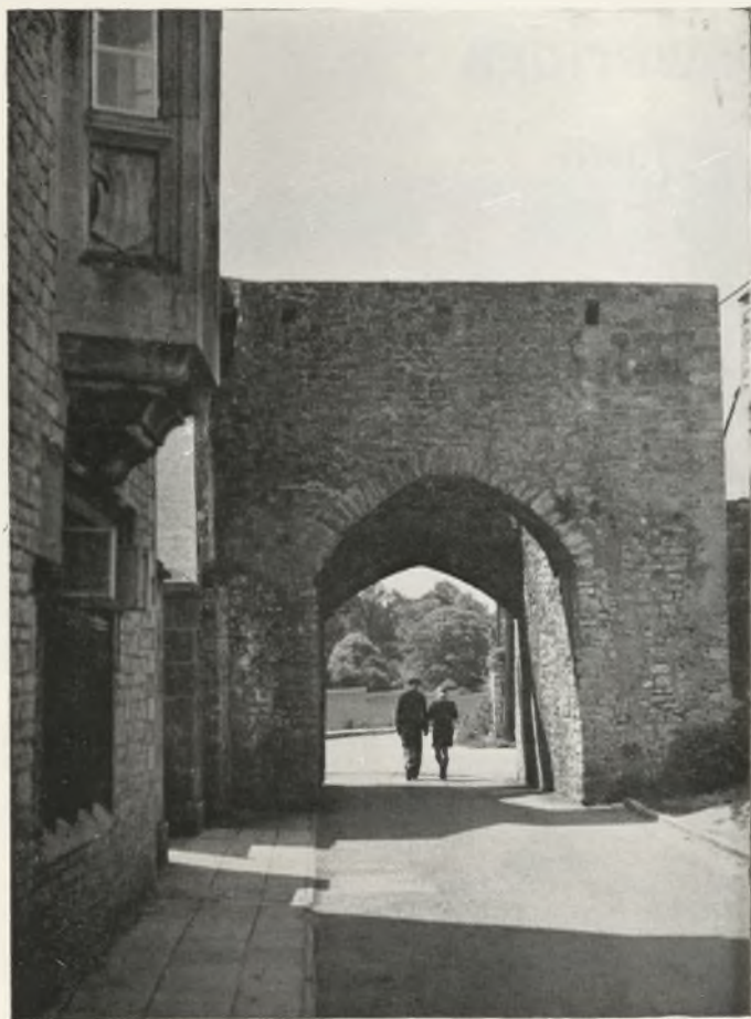
"PORTE MELIN", SOUTH GATE, TOWN WALLS, COWBRIDGE Ernest Carver & Son Ltd., Rvidgend
