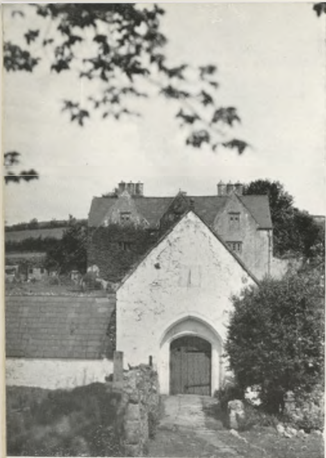
ABERTHIN TY MAWR BRIDGE GATE HOUSE Ernest Carver & Son Ltd., Bridgend
